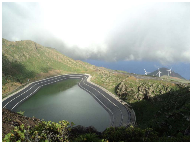
Fig. 3. Gorona del Viento, a hydro-wind energy plant in El Hierro Biosphere Reserve. Photo: Alba Juárez Bourke.
